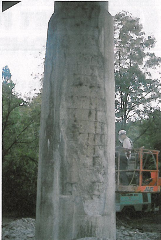
A badly deteriorated bridge pier
