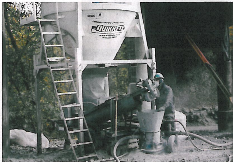
A material hopper with the material being predampened and fed into a rotary gunite machine during shotcrete placement
