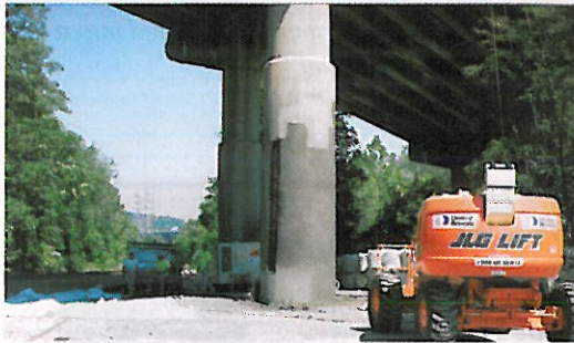
A shotcreted section of a bridge pier
