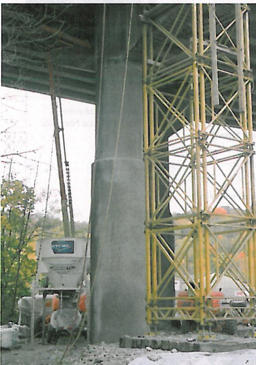
A completed shotcrete repair of a pier
